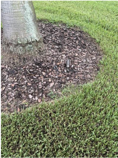
Fixture lying loose within the palm bed.
